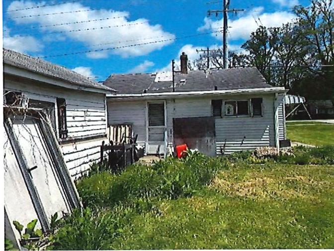
Figure 2 Rear view of 9023 Cincinnati-Dayton Road
