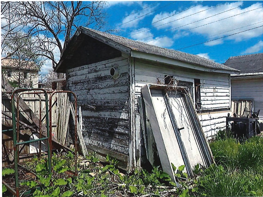
Exhibit D1.3 – Auxiliary Structure (Garage)
