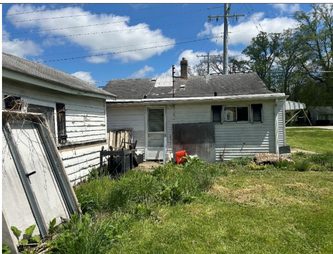
Figure 2 Rear view of 9023 Cincinnati-Dayton Road
