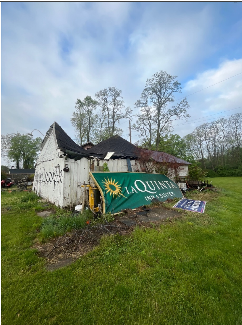
Figure 4 Garage located at 9031 Cincinnati-Dayton Road
