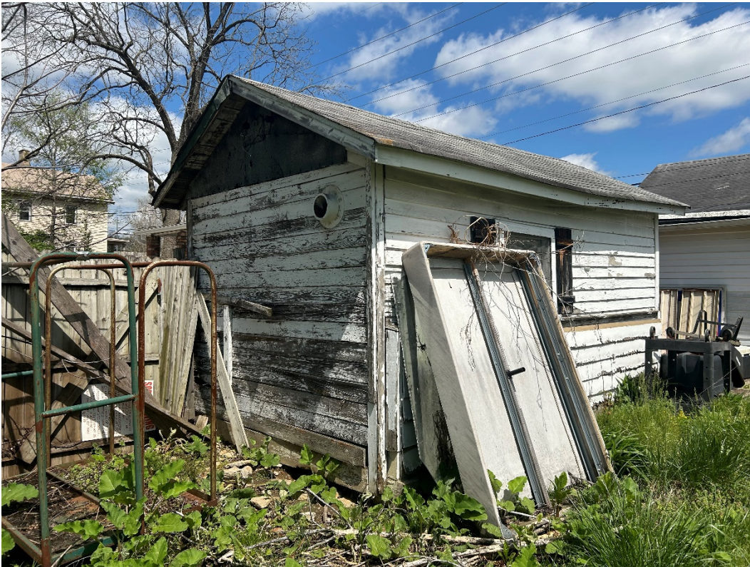
Exhibit D1.3 – Auxiliary Structure (Garage)
