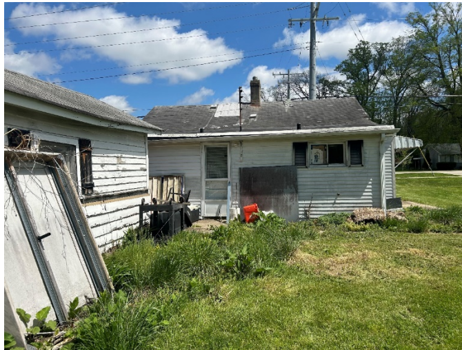
Figure 2 Rear view of 9023 Cincinnati-Dayton Road
